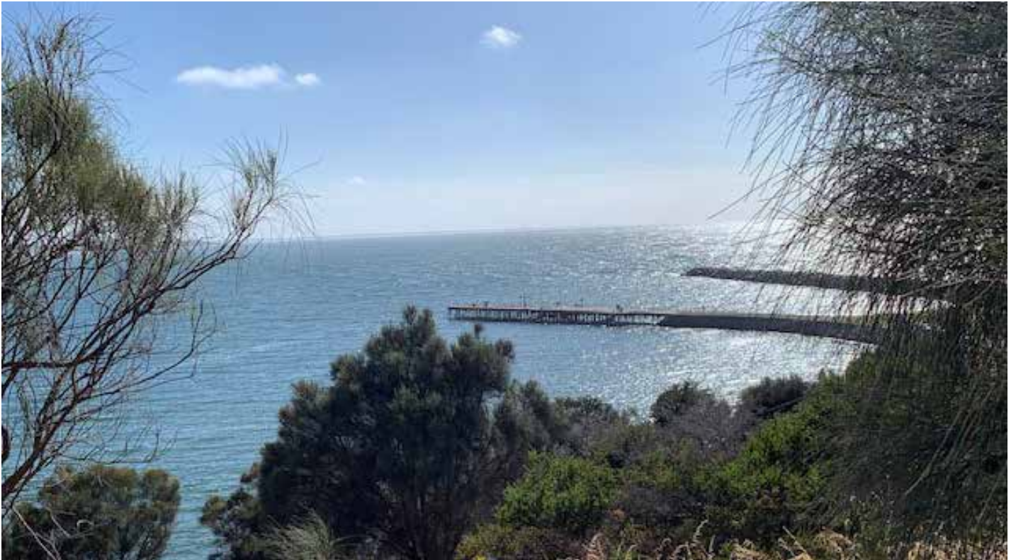
Screwpile jetty and breakwater from Granite Island
